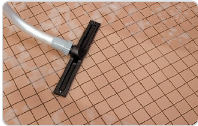
Soils and contaminants are vacuumed from the floor leaving the area clean and dry.
