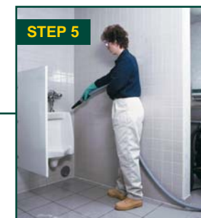
STEP 5 Blow dry surfaces & fixtures with separate blower hose and tool.
